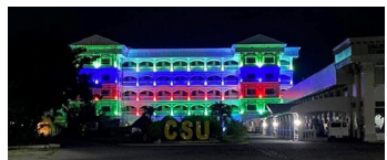
COMPLETION OF 5 STOREY CBEA BUILDING AT CSU ANDREWS
