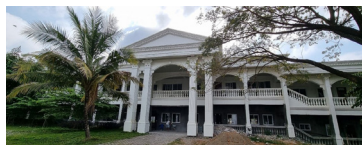
CONSTRUCTION OF CAS BUILDING A AT CSU CARIG Percentage Completed: 100%
